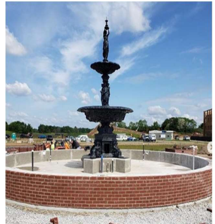
Robinson Iron fountain install, Louisville, KY.
