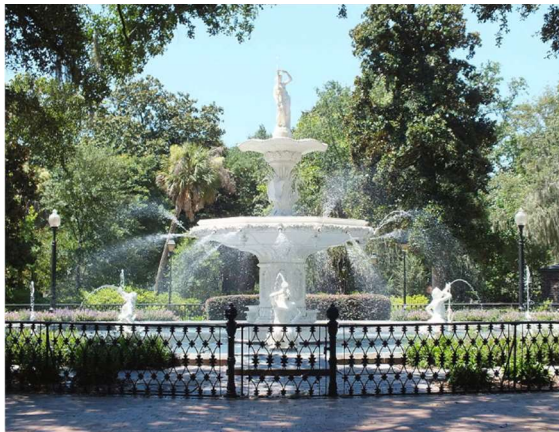
Repaired Forsyth Fountain, Savannah, GA.
