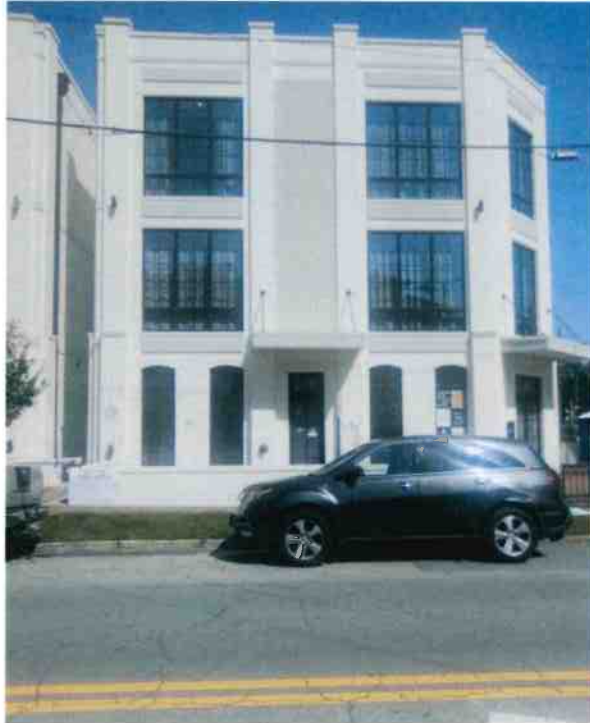
Front of Building
