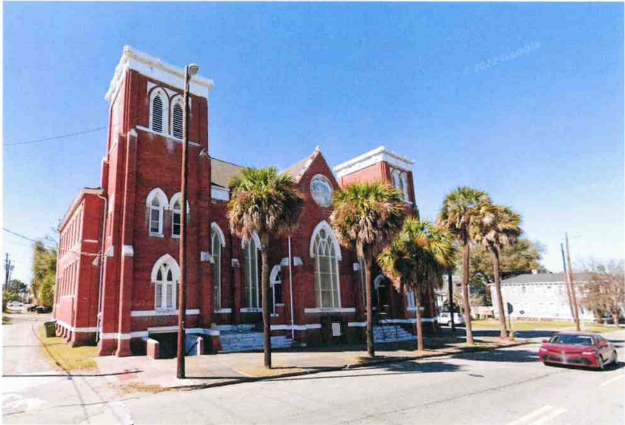
Figure 1: The current condition of the subject property.
