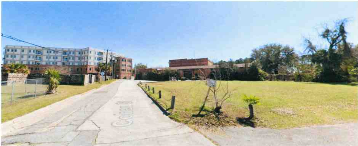
A view of Savannah Station and The Blake from the site proposed for development on Cohen St (right).
