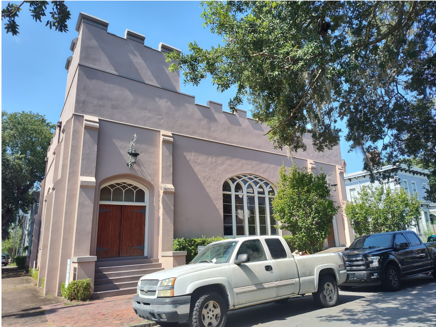
115 West Bolton Street
