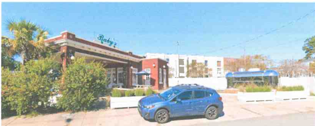
410 East 37 th Street - Site Conditions in 2026 (View from Price Street)
