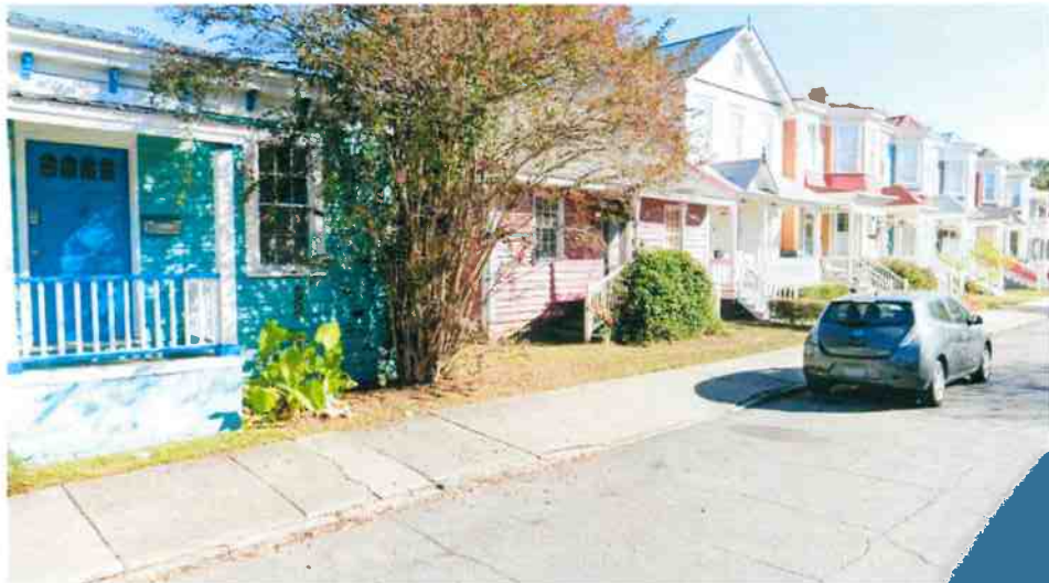
Facing North on E 41 st Street
