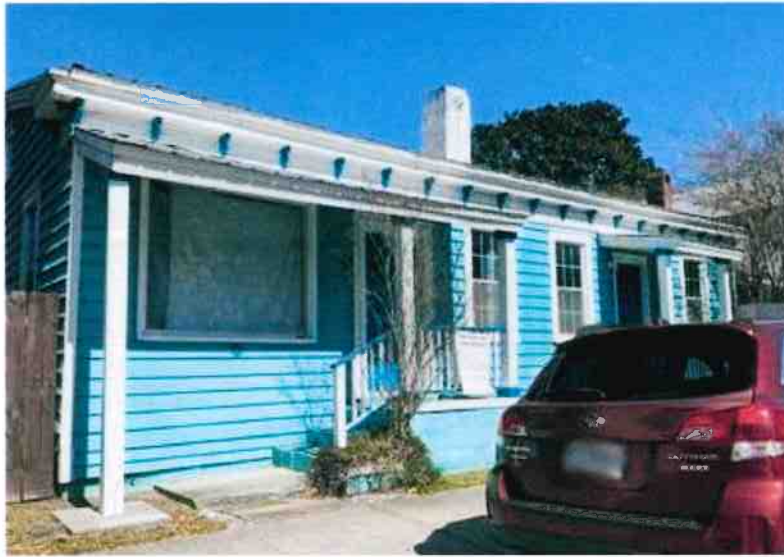
Photo of existing single-family residential building at 10 East 41 st Street
