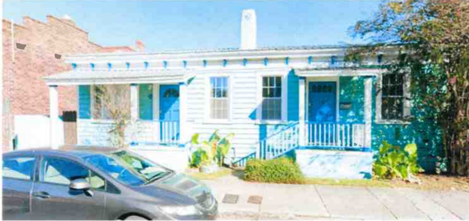
Front of building facing North on E 41 st Street
