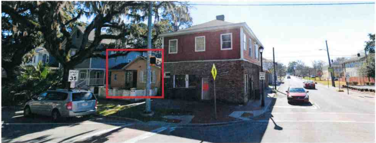
Existing dwelling on the property (yellow)
