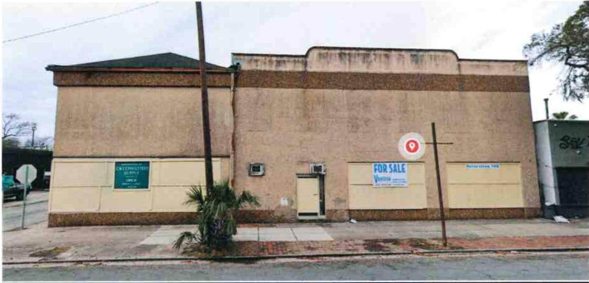
Existing Structure at 2517 Bull Street
