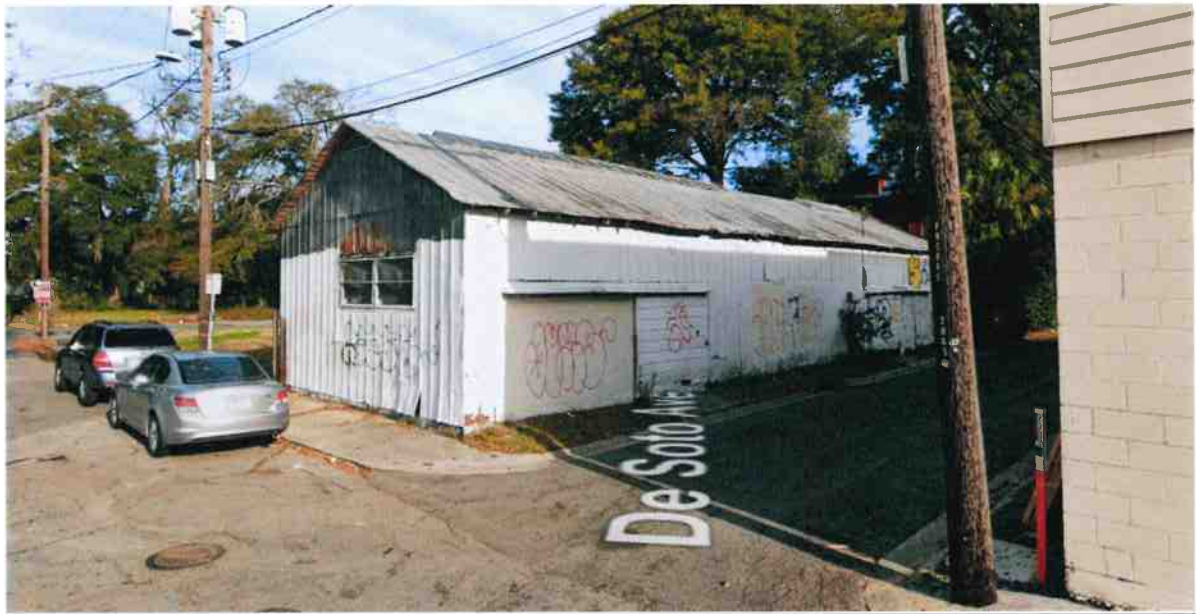
Existing Structure at 2517 W 42 nd Street
