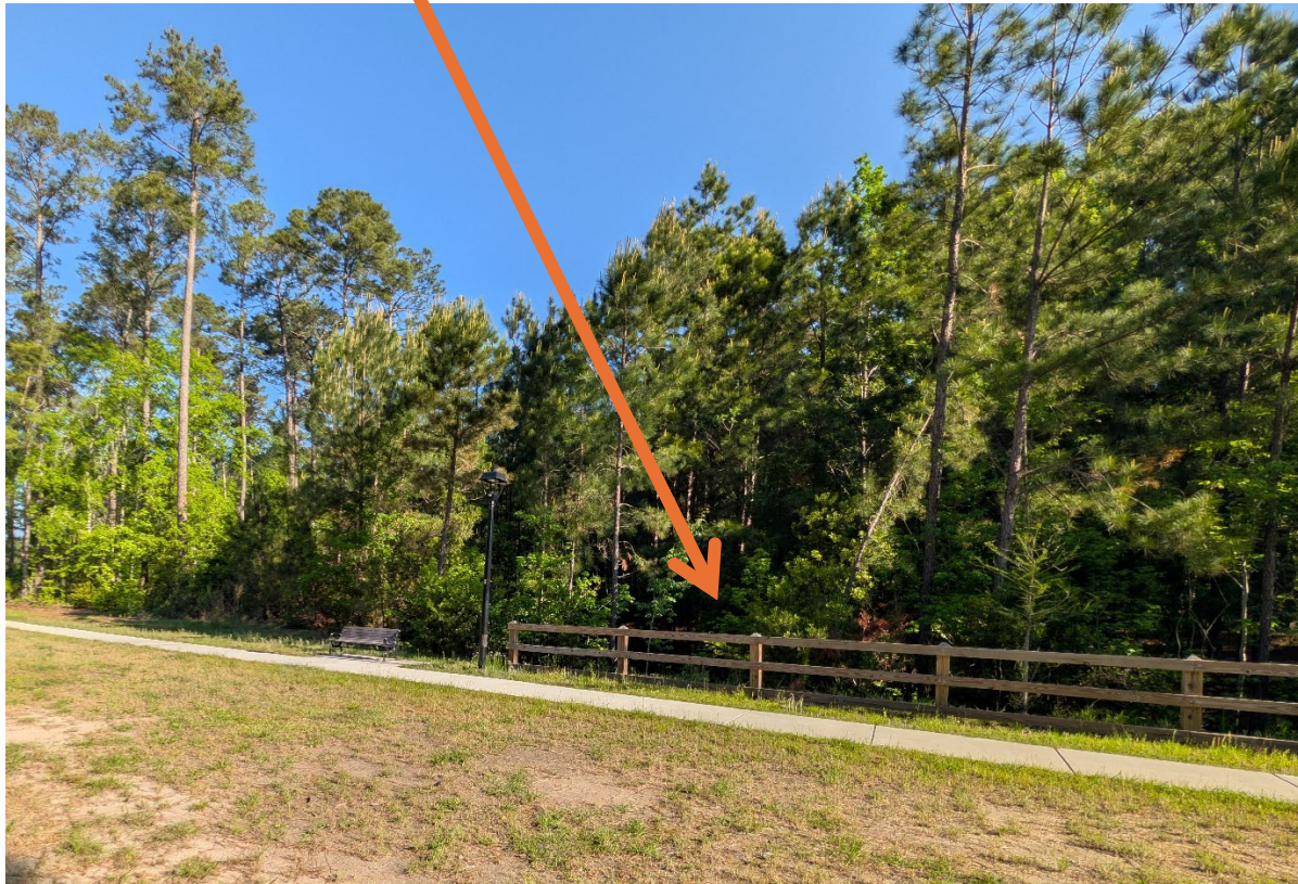
Drainage View Wide (F/N)
