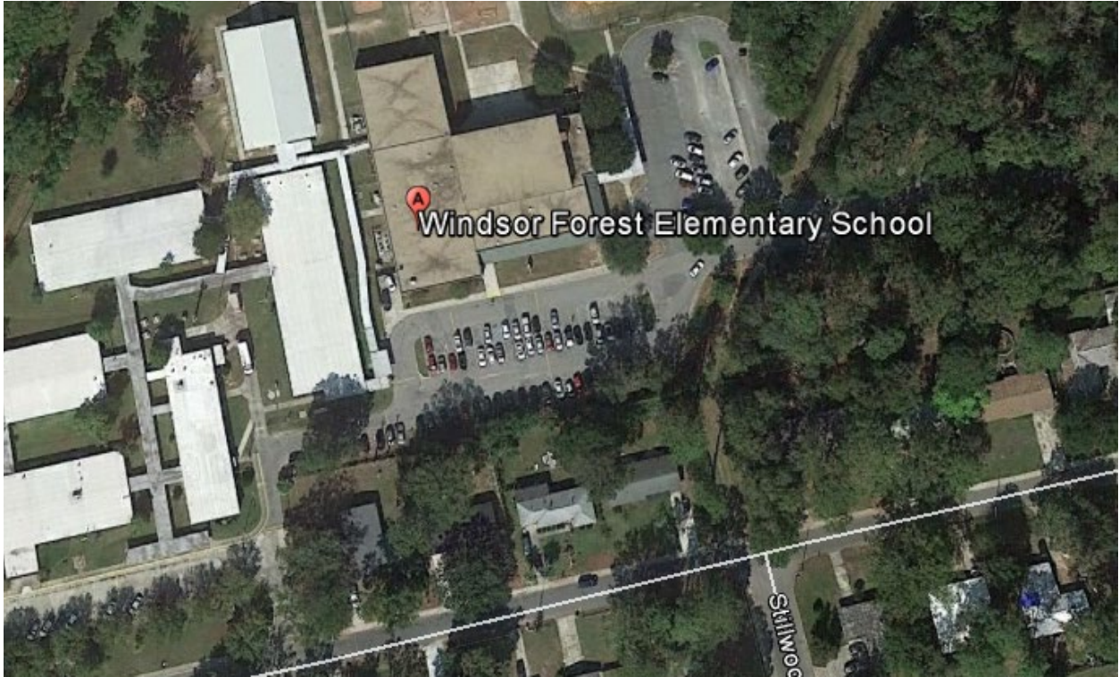
Windsor Forest Elementary School
