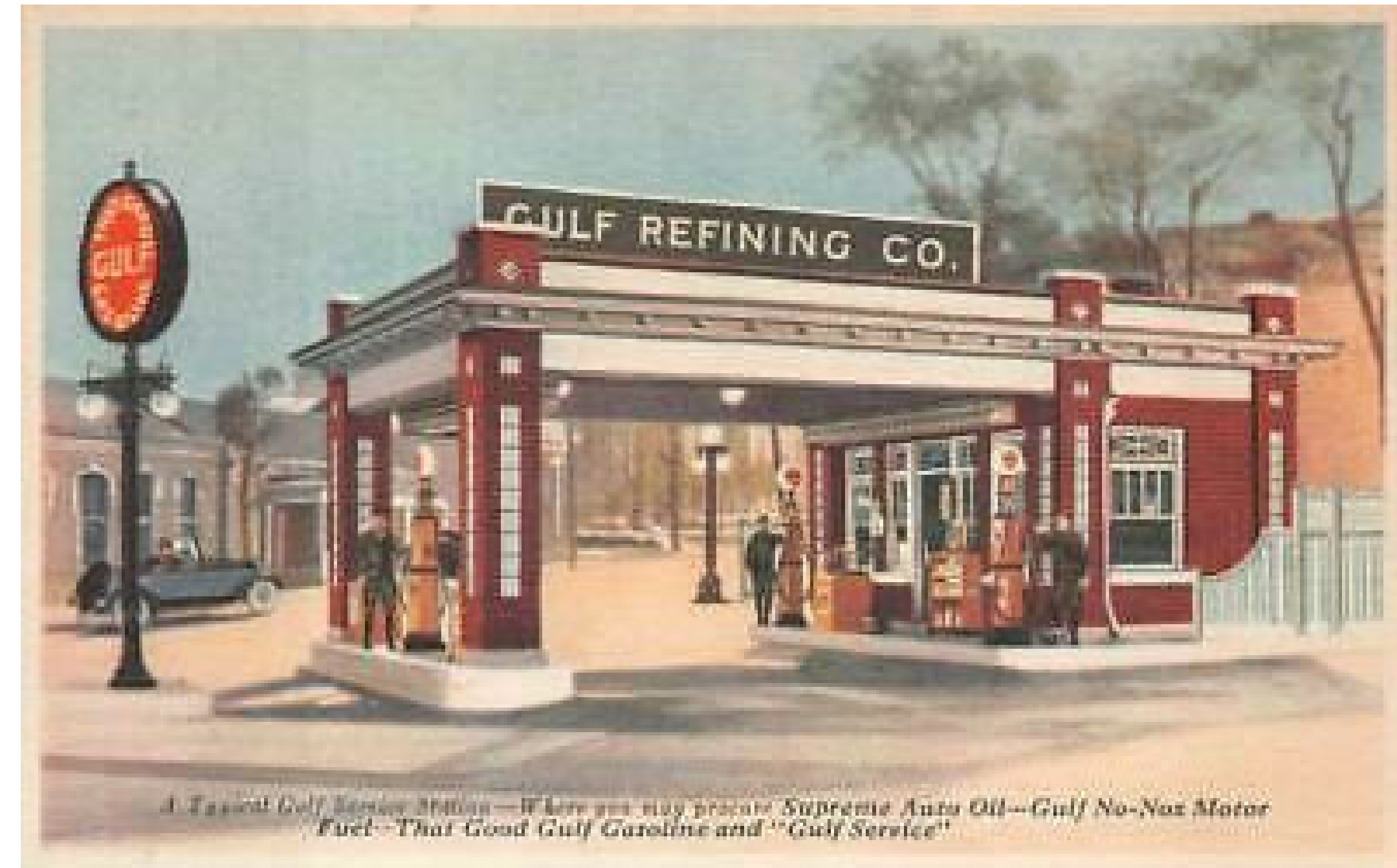
DETAILS ARE CONSISTENT WITH CEXISTING BUILDING AND OTHER EXISTING HISTORIC GULF STATIONS WITHIN REGION.
