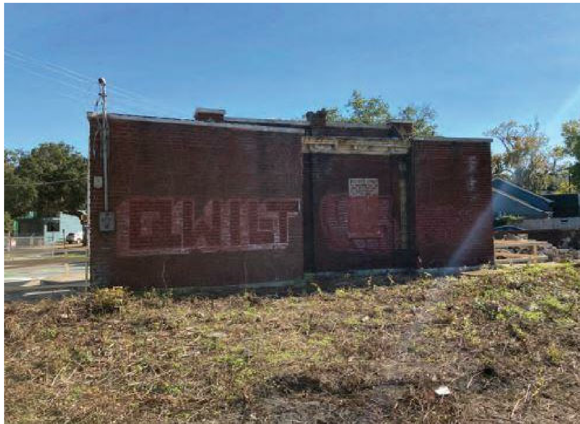
REAR ELEVATION - FACING RAILROAD TRACKS
