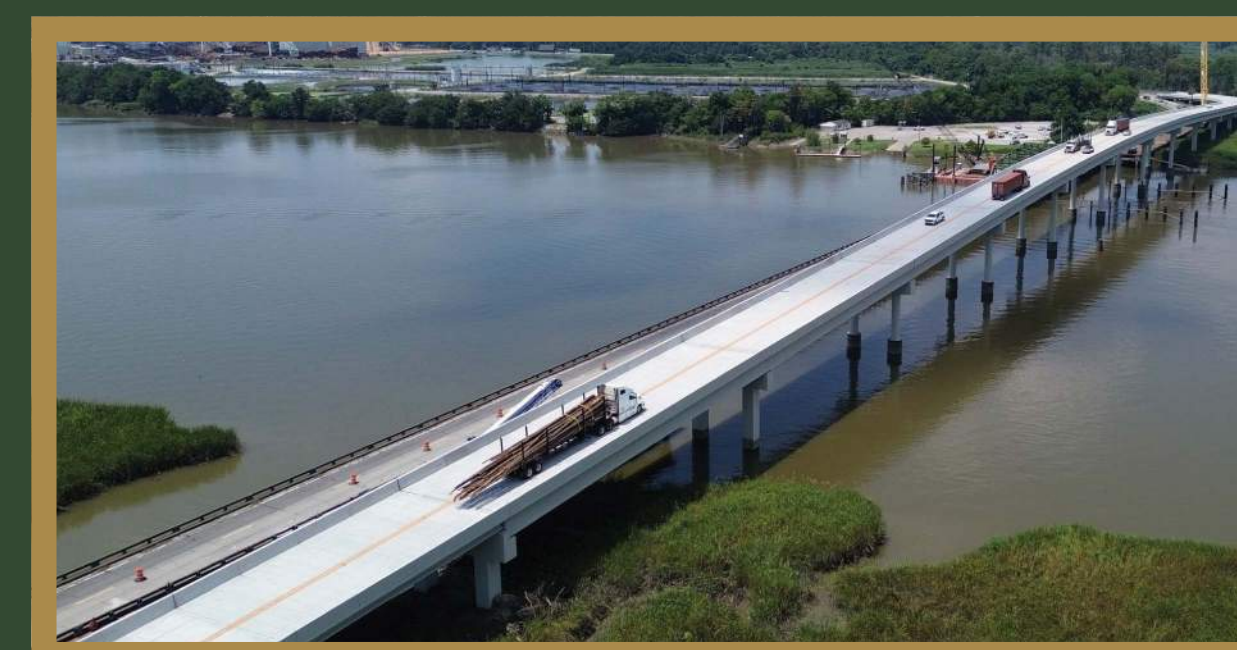
New Houlihan Bridge in 2025
