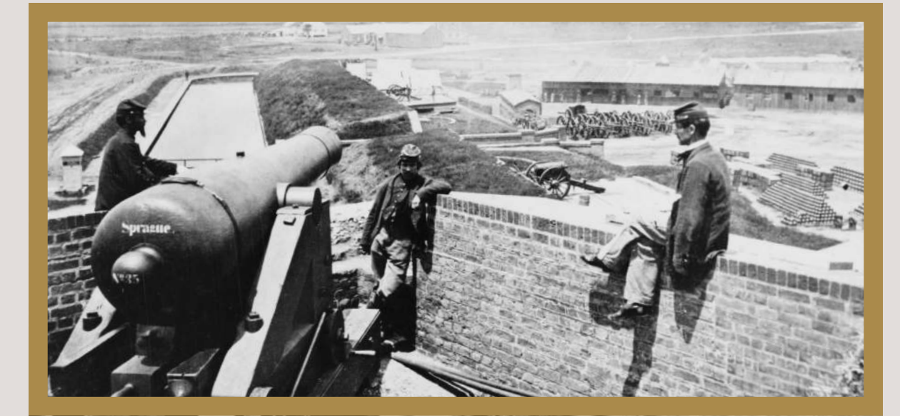
Southwest corner of Fort Pulaski, 1863
