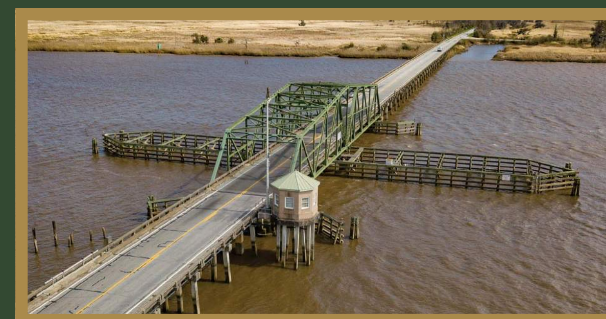
Houlihan Bridge in 2021
