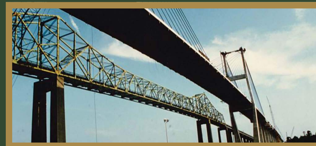
Construction of the Talmadge Bridge in 1991 Courtesy Georgia Historical Society
