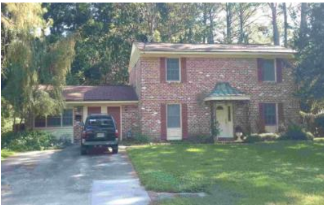
Slab-on-grade house with no gutters and a drainage inlet in front yard
