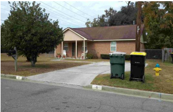
Slab-on-grade house with ground level HVAC unit
