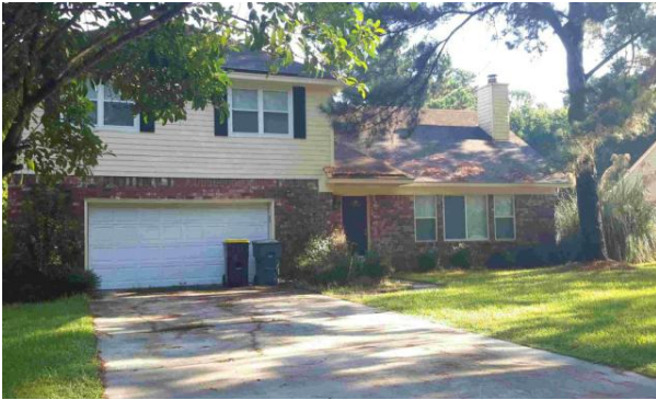
Slab-on-grade house with no gutters
