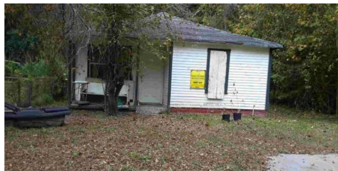
Vacant single-story building in poor condition
