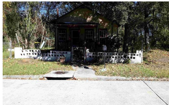
House with curbs and drainage inlet located in front yard
