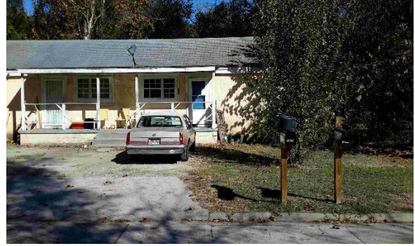
Multi-family duplex with a raised slab-on-grade foundation
