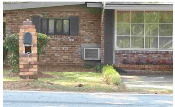
Single story house with HVAC attached to masonry a few feet off the ground
