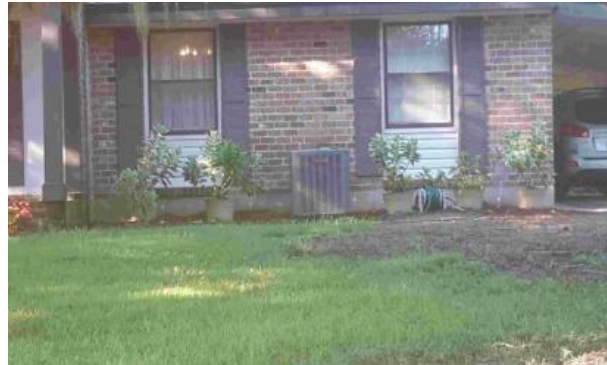
Single family residence with no gutters and HVAC located at ground level
