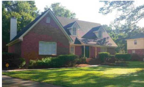
Two-story house with crawl space and HVAC unit located at ground level
