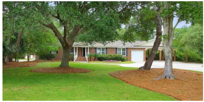
House with elevated crawlspace
