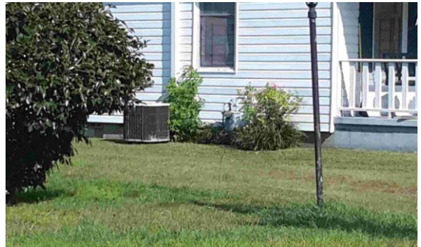
House with HVAC unit at ground level
