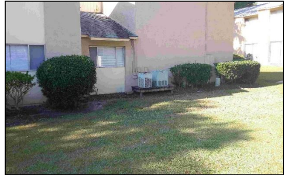
Multi-family townhomes with slightly raised HVAC system
