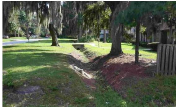
Single family residential home with culvert running through front yard
