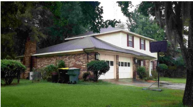
Slab-on-grade house with HVAC located on ground level
