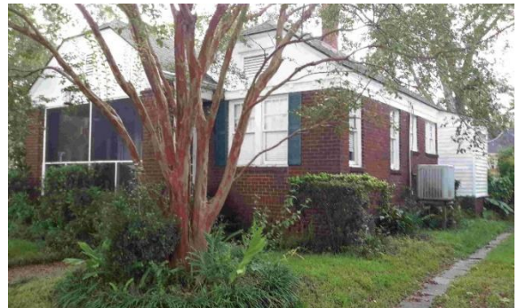
Single family home with HVAC raised to first floor
