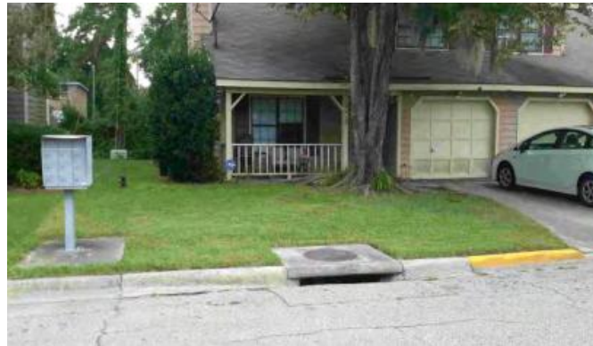
Multi-family condos with no gutters and a drainage inlet in the front yard
