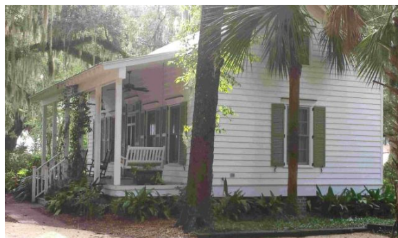
House elevated on 3-4-foot tall brick columns
