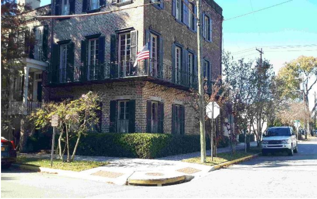
At grade residential building with drainage inlet and curbs located on corner
