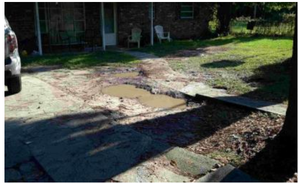
Yard with signs of flooding
