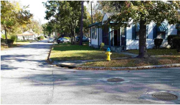
Slab-on-grade house with no gutters and a drainage inlet on the corner
