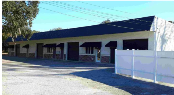
Commercial building with large impervious parking lot
