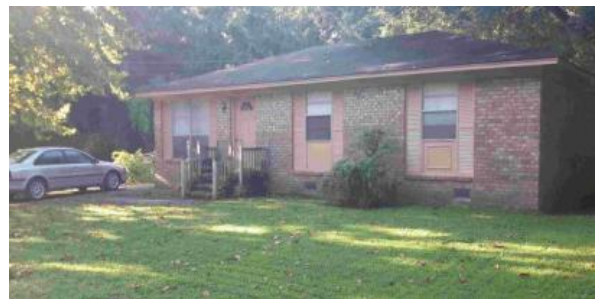
Home with a crawlspace foundation and no gutters
