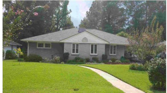
House with crawlspace foundation and ground level HVAC
