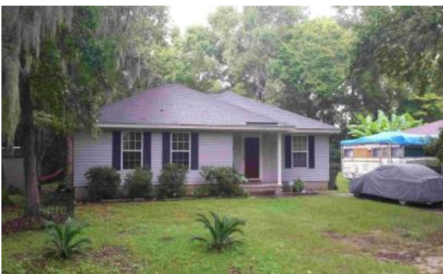
Slab-on-grade house with no gutters that sits next to a small creek
