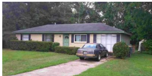
Slab-on-grade house with ground level HVAC unit
