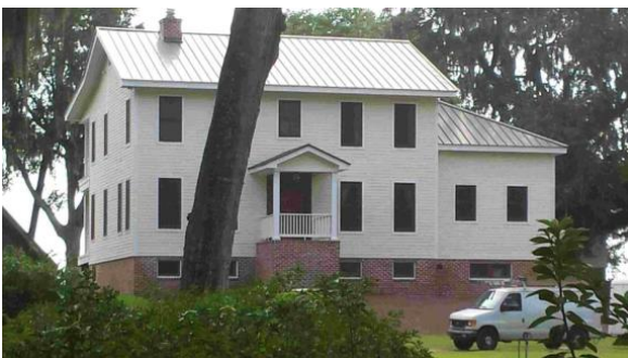
Two-story house with an enclosed elevated foundation
