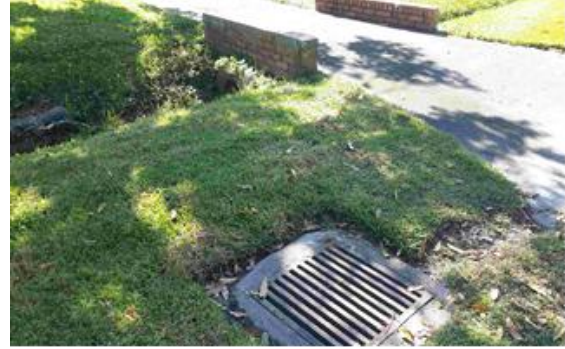
Single family residential lot with drainage ditch and inlet located in front yard
