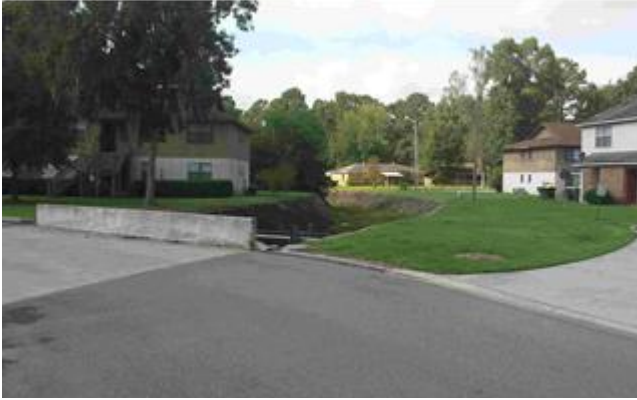
Multi-family townhomes with large drainage ditch running between structures
