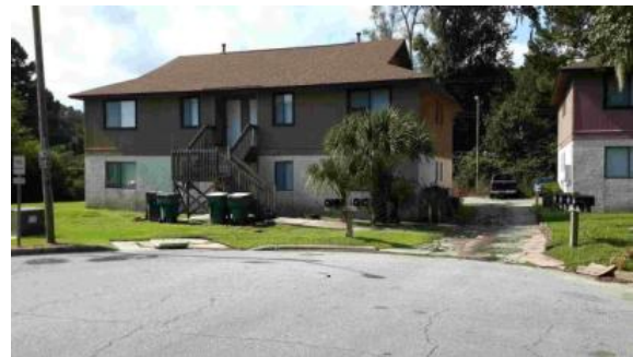
Multi-family apartment building with curbs and drainage inlet located in front yard
