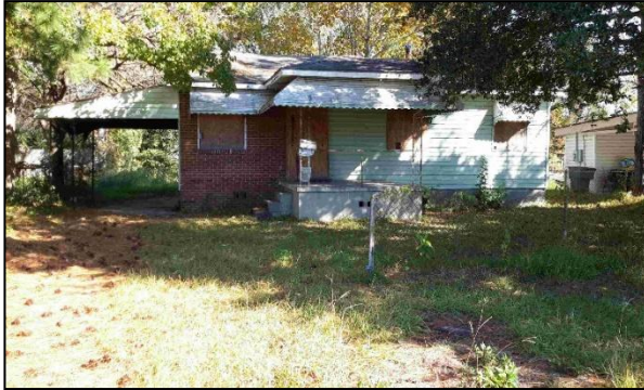
Abandoned house with repairs needed
