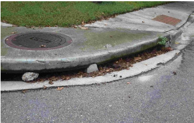
Stormwater drainage inlet
