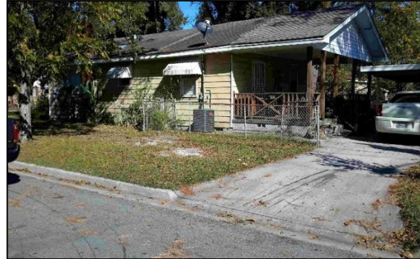
House with a crawlspace foundation type and an HVAC unit at ground level
