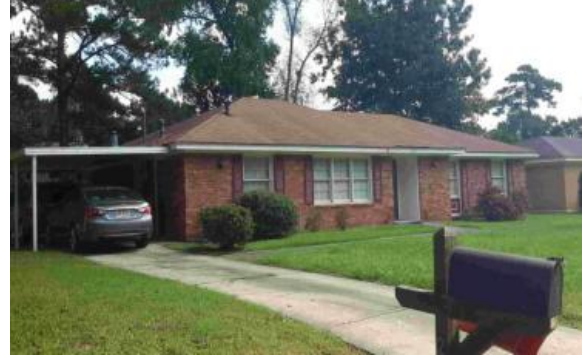
Slab-on-grade house with no gutters and ground level HVAC unit
