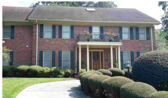
Two story house with a crawlspace foundation and gutters
