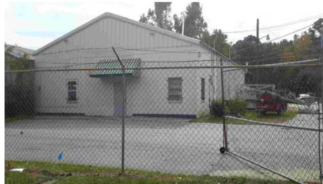
Commercial building with large impervious parking lot and no gutters
