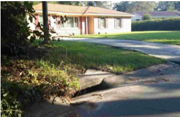
Slab-on-grade home with no gutters and a stormwater inlet located near driveway
