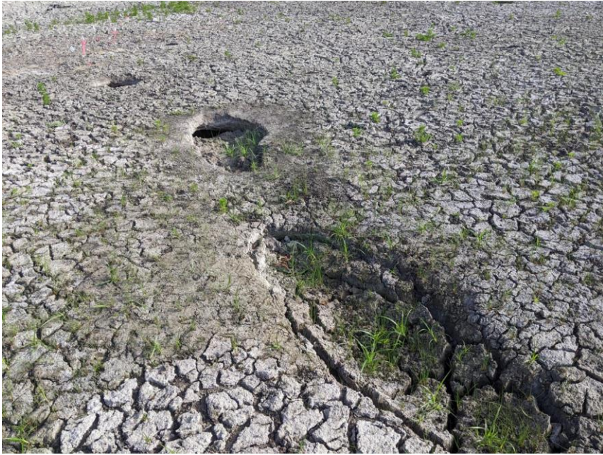
Holes in the bottom of the pond formed a network of water exiting points
