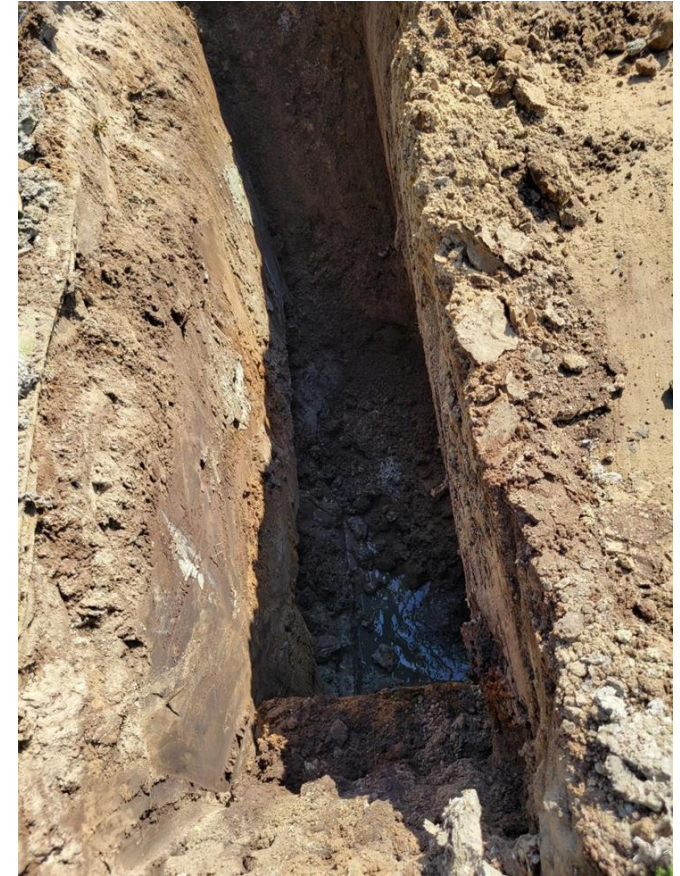
Void at more than 5 feet in depth and goes below the embankment
