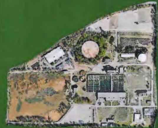
Site clearing, dredging, chemical storage & utility relocations
