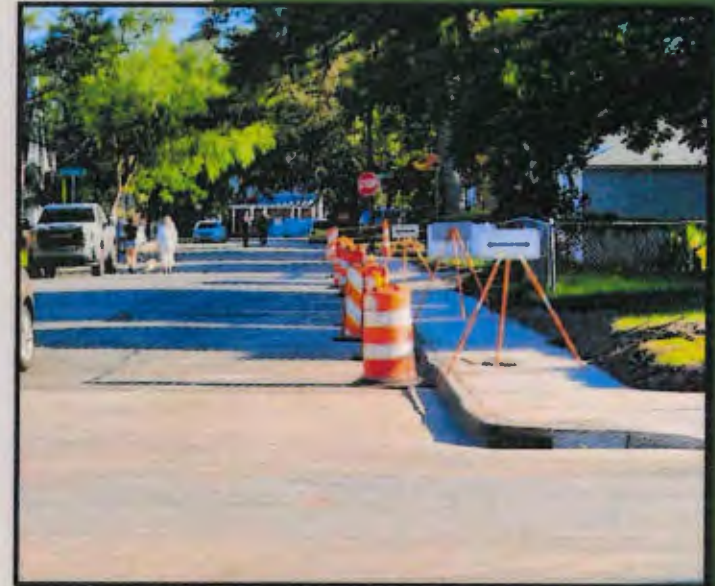
Batley Street Sidewalk Construction
