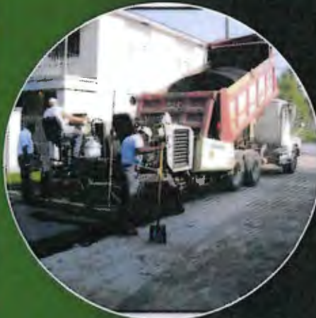
Resurfacing work in Savannah
