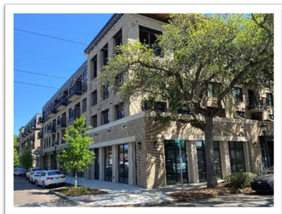
New market rate apartments constructed fronting E 31 st Street between Bull and Abercorn Streets
