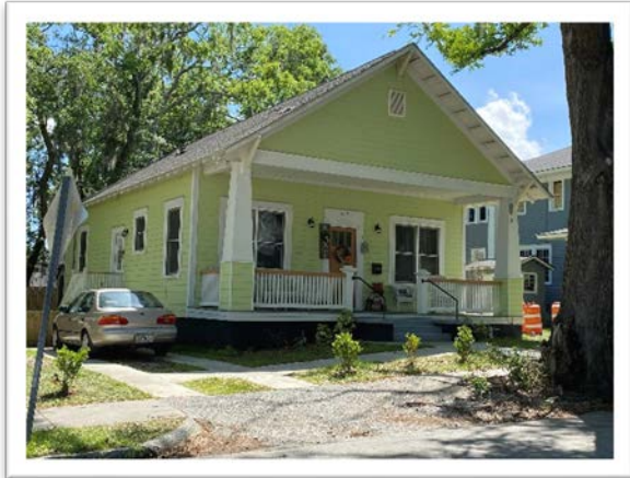
New single-family house built and sold to a first-time low-income home buyer by Habitat for Humanity in partnership with the City.
