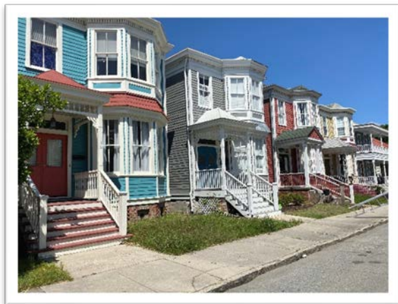
Historic 2-story houses once deteriorated and vacant now renovated in the first block of E. 41 st Street
