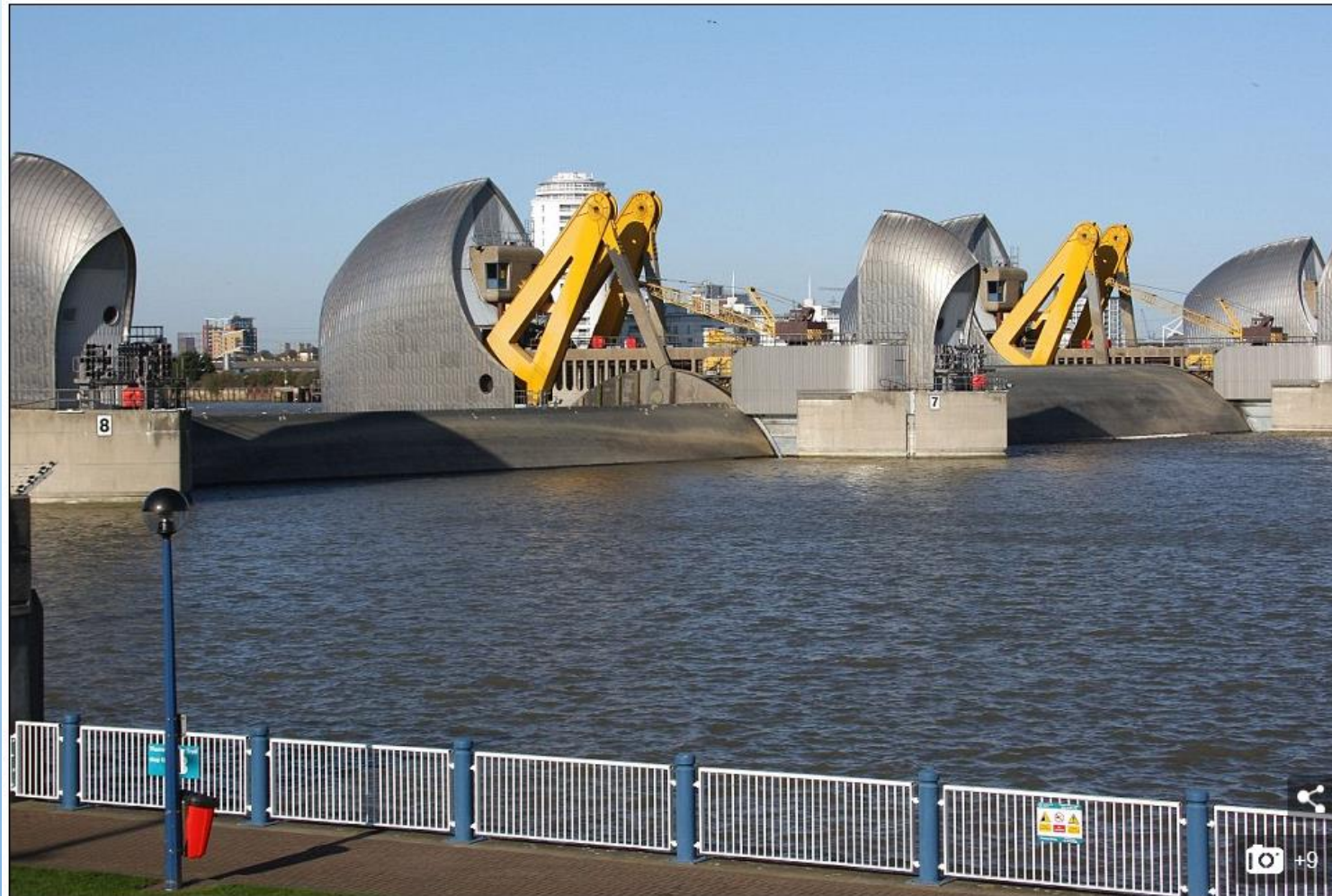
The Thames Barrier (pictured in action), which is operated by the Environment Agency, has 10 steel gates that can be raised into position across the River Thames. When raised, the gates stand as high as a five-storey building and as wide as the opening of Tower Bridge
