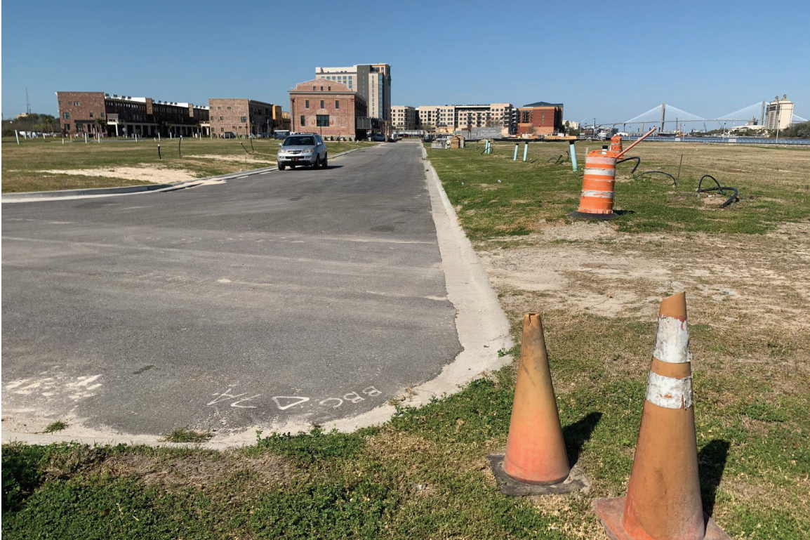
Viewing East along the northern most paved road within the Eastern Wharf project from the southern end of the proposed access easement.
