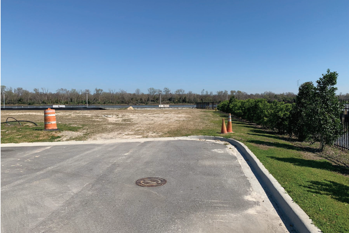
Viewing North toward the Savannah River from the current limits of paved access across the proposed access easement and R/W # 1 and #2.
