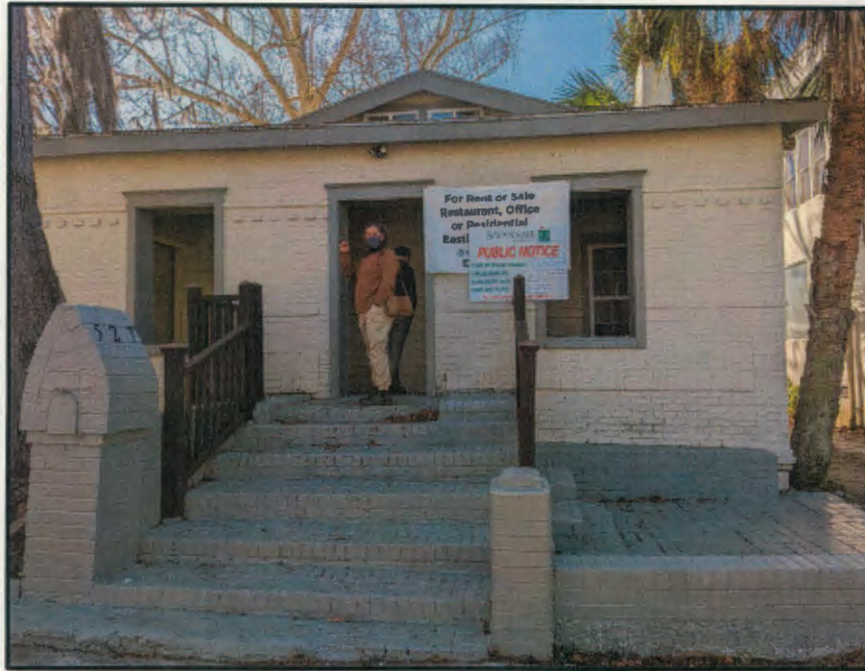
Front of the building that will be used for the daytime café and the nighttime restaurant.
