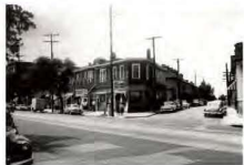
The corner of West Broad Street and Roberts Street, shortly before demolition for the I-16 exit ramp.
