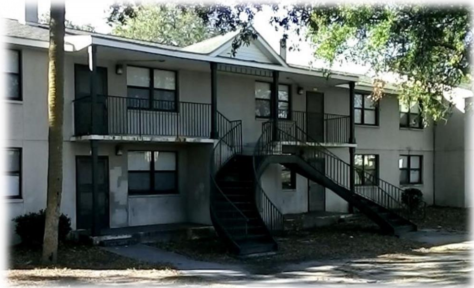
Former Fred Wessels site
