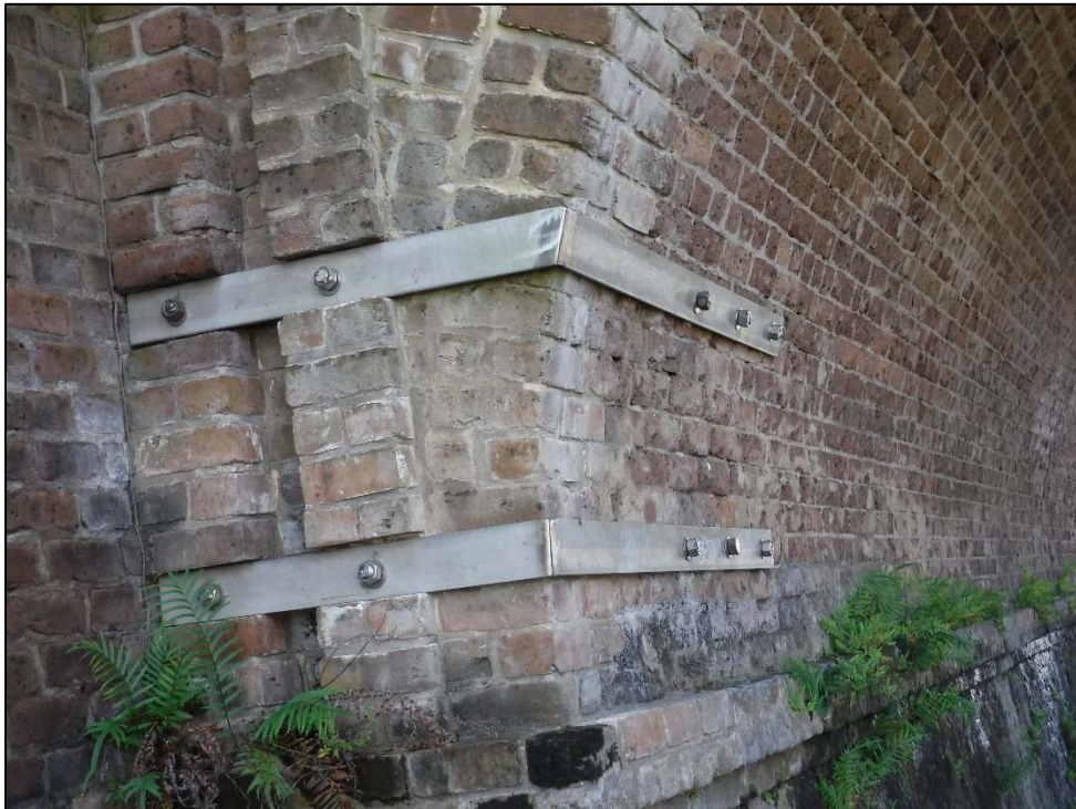
Photograph 44 – Stainless Steel Brackets at Arch 4
