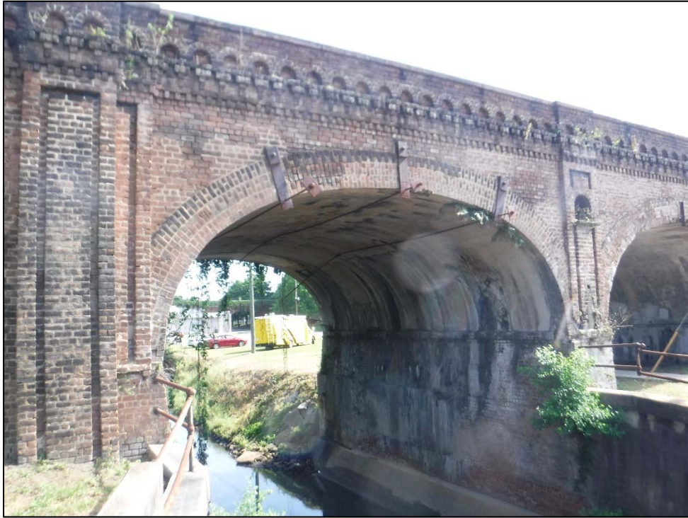
Photograph 7 – Arch 1 Looking Northeast
