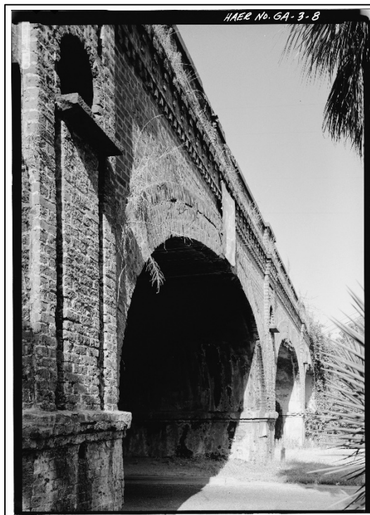
Photograph 8 – Arch 2 Looking Northeast
