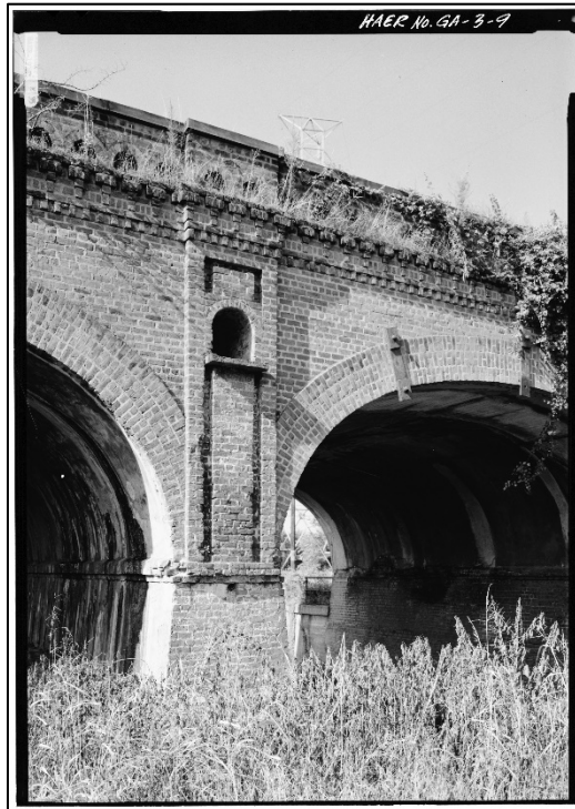
Photograph 9 – Arch 3 Looking Northeast
