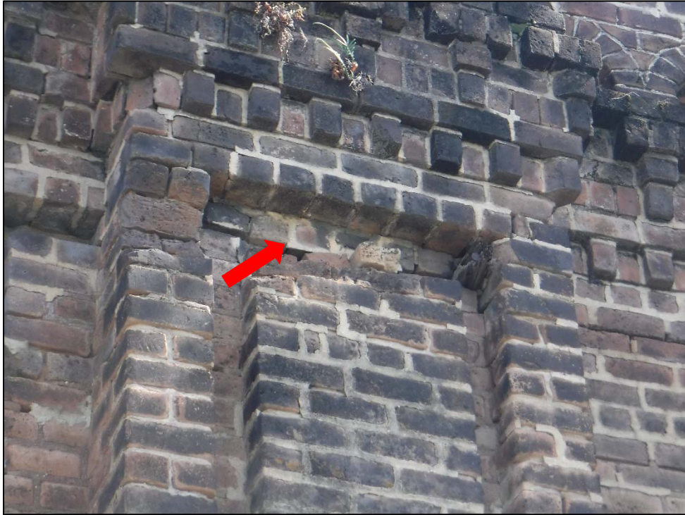
Photograph 63 – Missing Bricks
