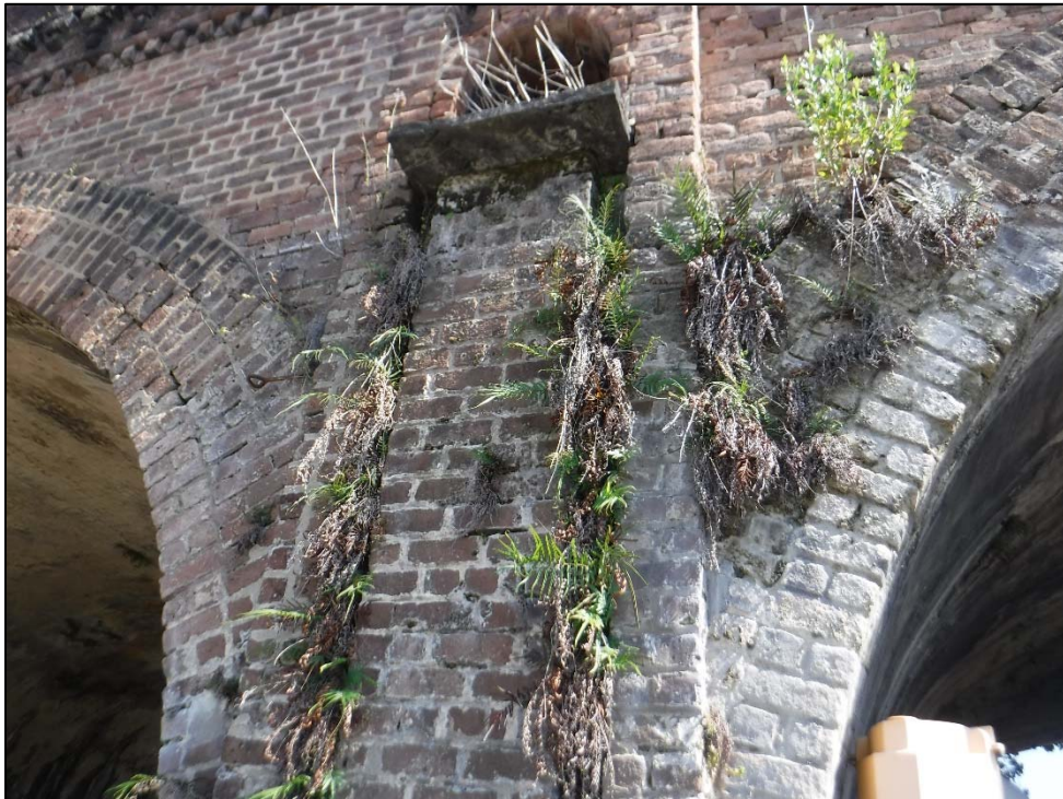
Photograph 60 – Vegetation Growth at South Elevation
