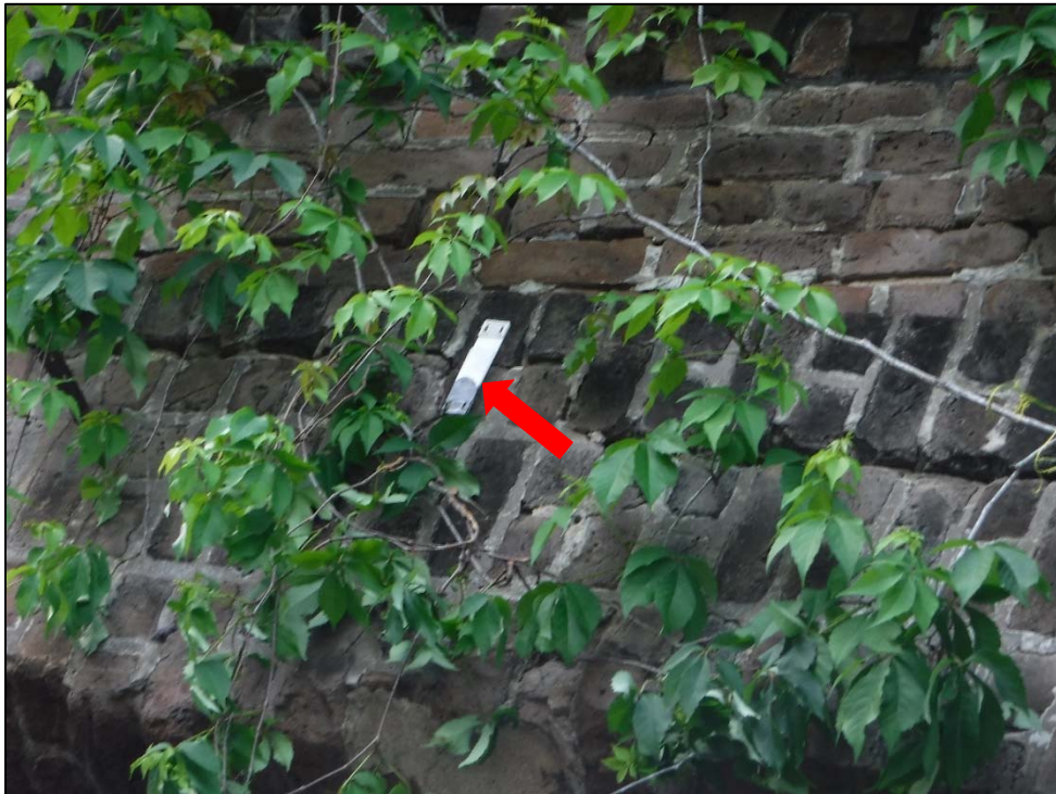
Photograph 40 – Crack Gauge at Arch 4
