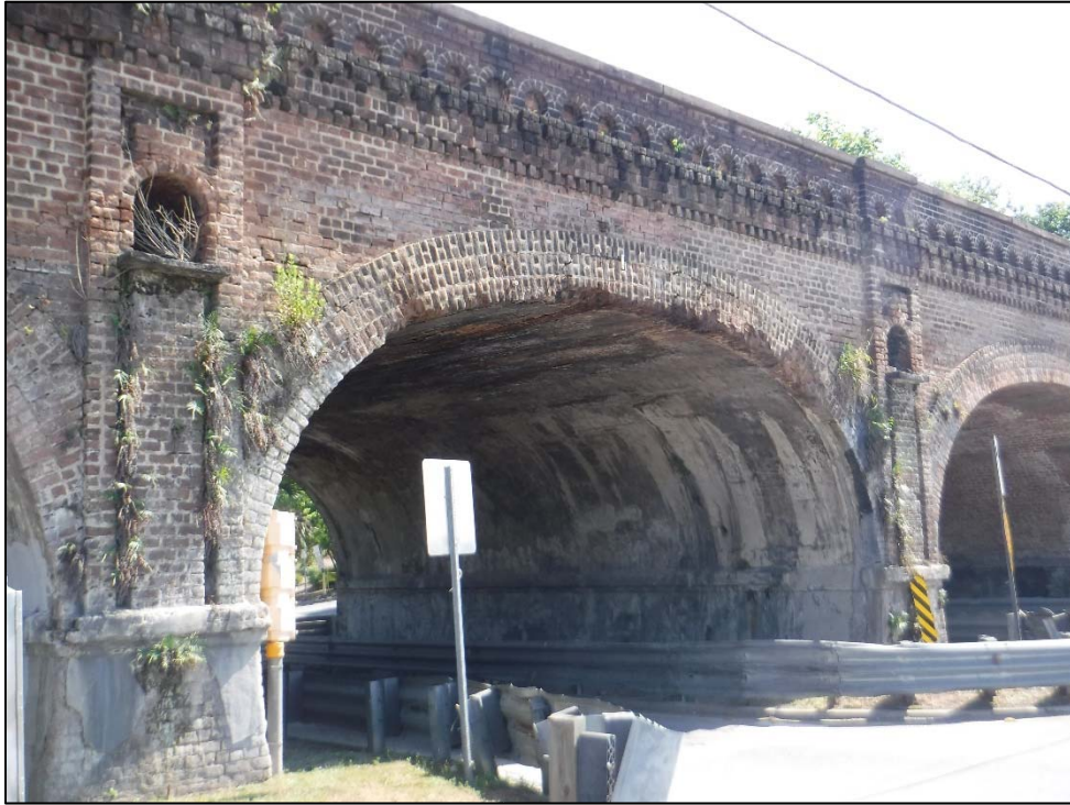
Photograph 9 – Arch 3 Looking Northeast
