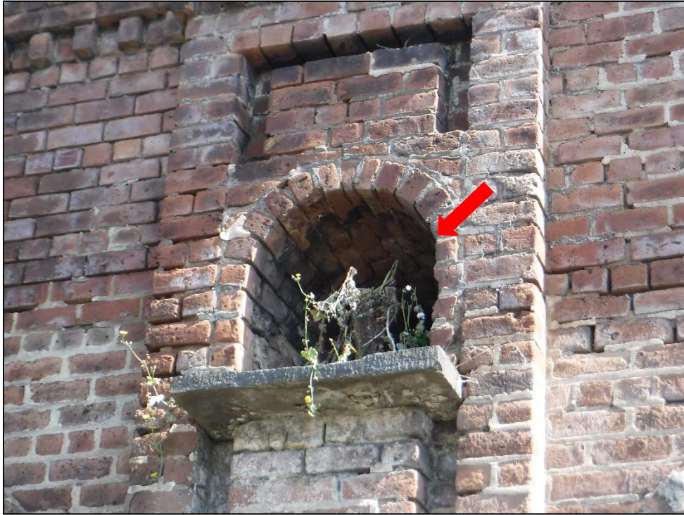
Photograph 13 – Typical Open Arch at Pier
