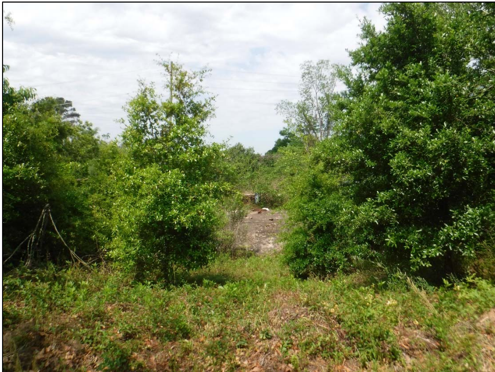
Photograph 4 - Viaduct from East Approach
