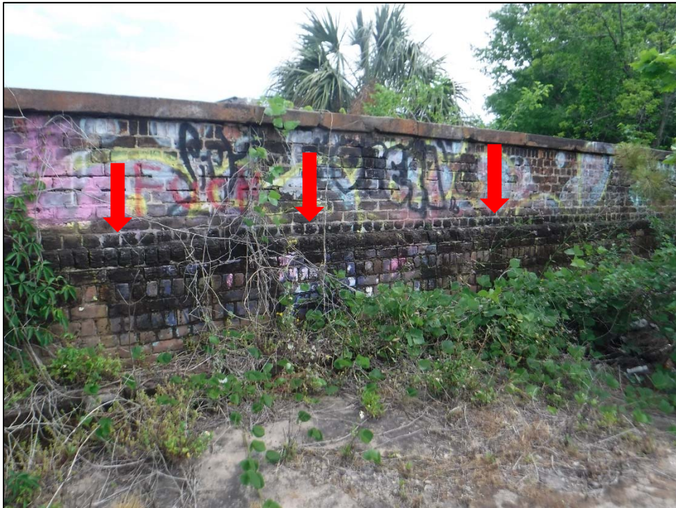
Photograph 20 – Fill Removed from Top of Viaduct
