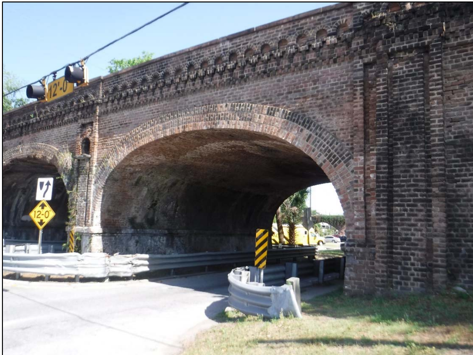
Photograph 10 – Arch 4 Looking Northwest
