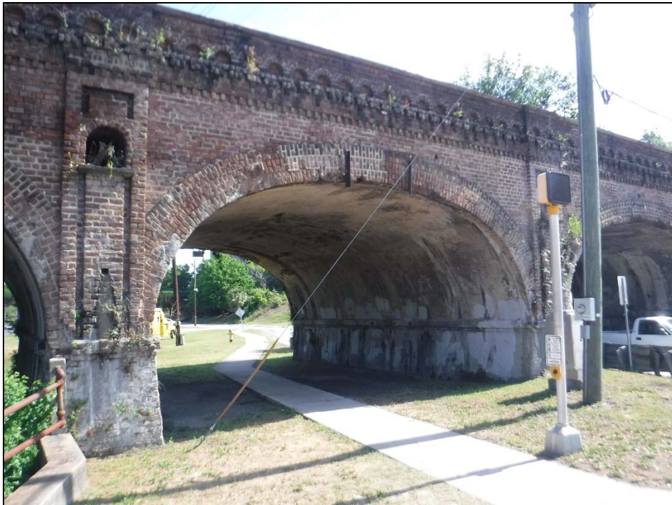
Photograph 8 – Arch 2 Looking Northeast
