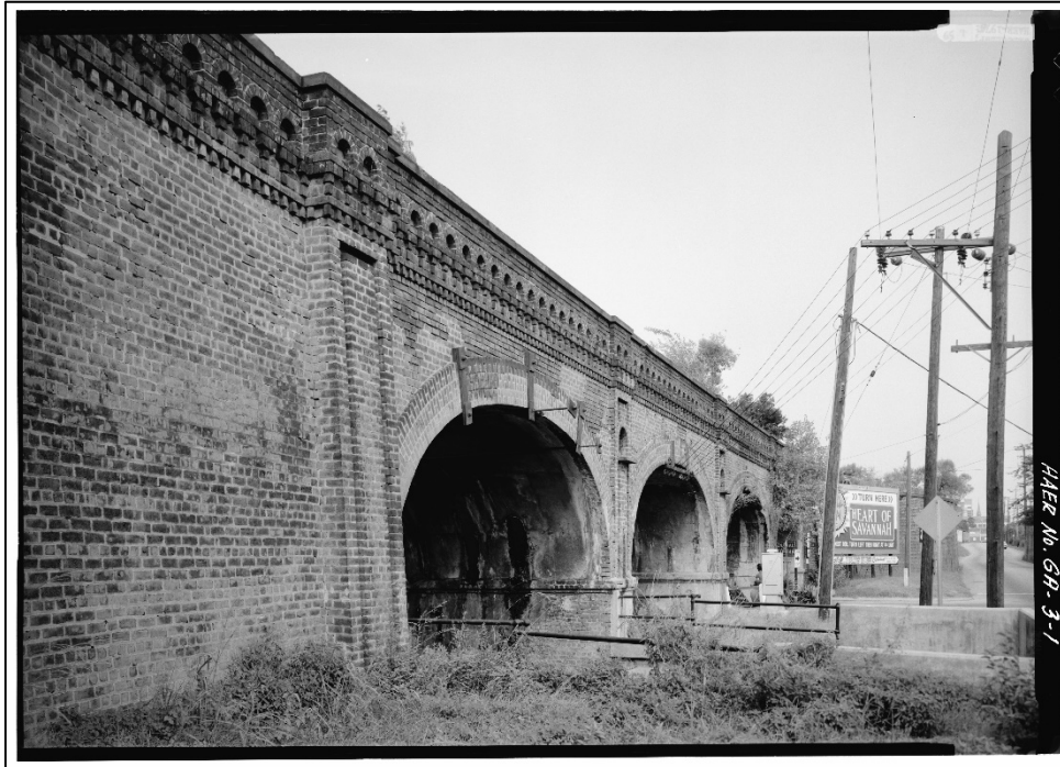
Photograph 1 - West Approach Looking West
