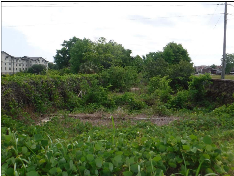
Photograph 2 - Viaduct from West Approach
