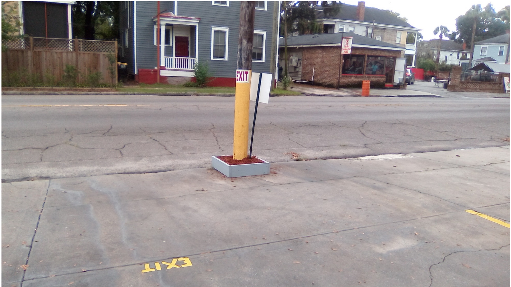
Exit signage with planters around a utility pole.
