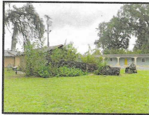
Rear of Property (South end) Stump and overgrowth
