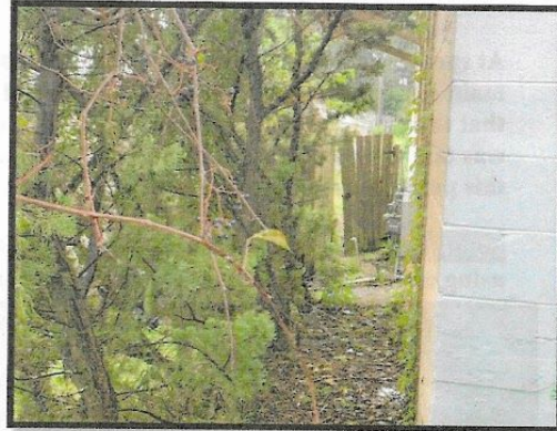
Rear of Building on the East behind rooms
