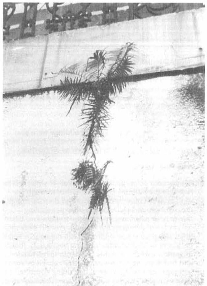
Fig. 12. (a) Water intrusion caused by rusting metal, or (b) plant growth left unattended will gradually enlarge these cracks, resulting in spalling, and eventually requiring extensive repair of the stucco. Photos: National Park Service Files.
