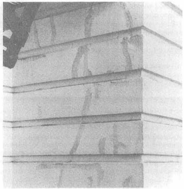
Fig. 13. (a) In preparation for repainting, hairline cracks on this Mediterranean style stucco apartment building were filled with a commercial caulking compound; (b) dirt is attracted and adheres to the texture of the caulked areas, and a year after painting, these inappropriate repairs are highly obvious. Photos: Anne Grimmer.
