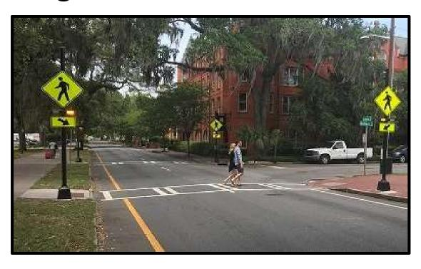
The Beacons and Pedestrian Pushbuttons were installed at 8 intersections next to Forsyth Park in an effort to improve pedestrian safety.
