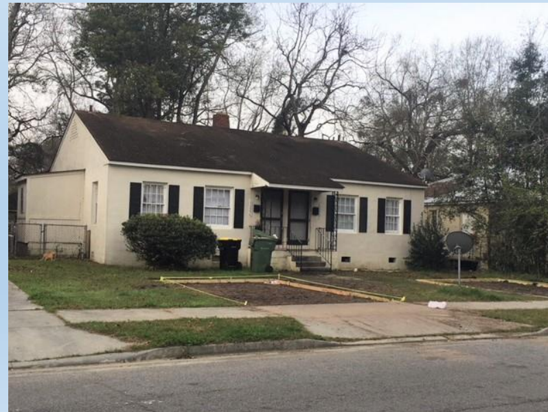
Top Right – Unsafe front yard parking before adoption of residential parking ordinance.
