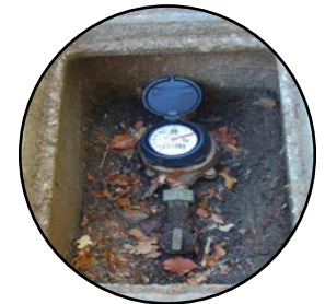
Water Meter Leaks
