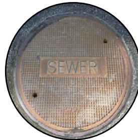
Sewer Maintenance Investigation
