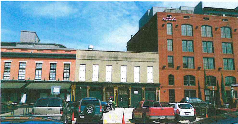
View of existing buildings located within the 2 stories above Bay Street and 3 stories above Bay Street as defined by the current height map allowance.
