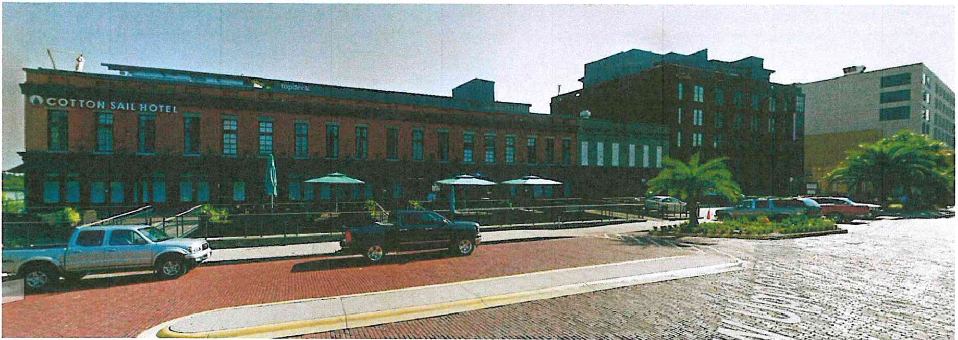
Existing buildings located between Barnard Street and Whitaker Street within differing allowable stories above Bay Street within Savannah Historic District Height Map.
